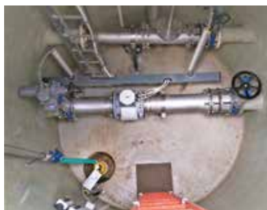
Electrical flow control, dry operation
