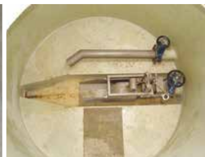
Mechanical flow control, semi-dry operation
