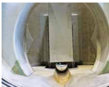
Left: Throttle valve without moving parts, wet well installation
