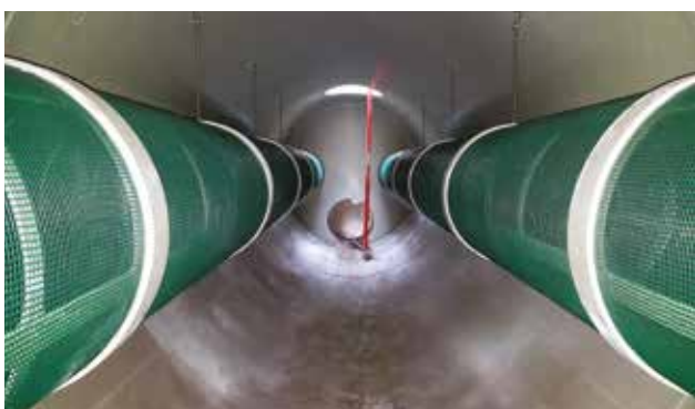
Storage sewer with Amiblu Amiscreen elements. The large screening surfaces effectively filter suspended solids from the wastewater.
