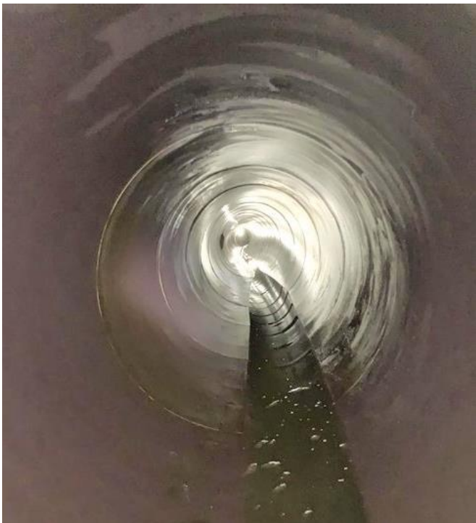
Fig 4: Restored pipeline ready for handover to Wessex Water
