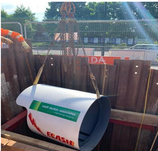
Fig 2: MDA Ltd works preparation
