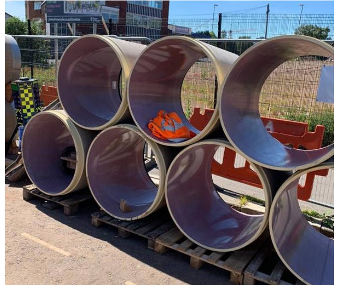
Fig 3: Amiblu DN900 Jacking Pipes
