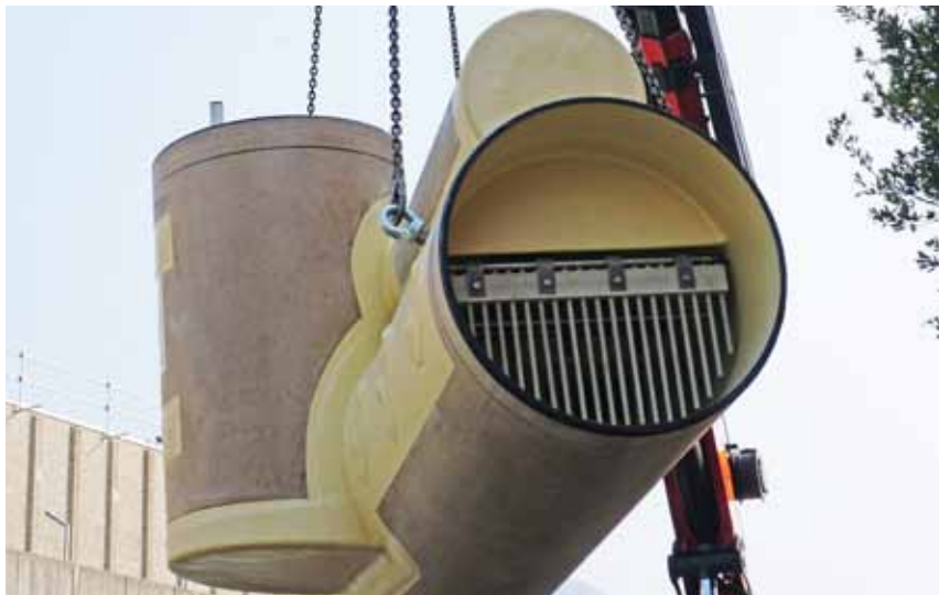
Top left: The CSO chamber was successfully installed in 1 day only. Bottom right: The highly effective and flexible cleaning elements (GRP bars). Top right: The project team did a great job and is pleased with the optimal result.
