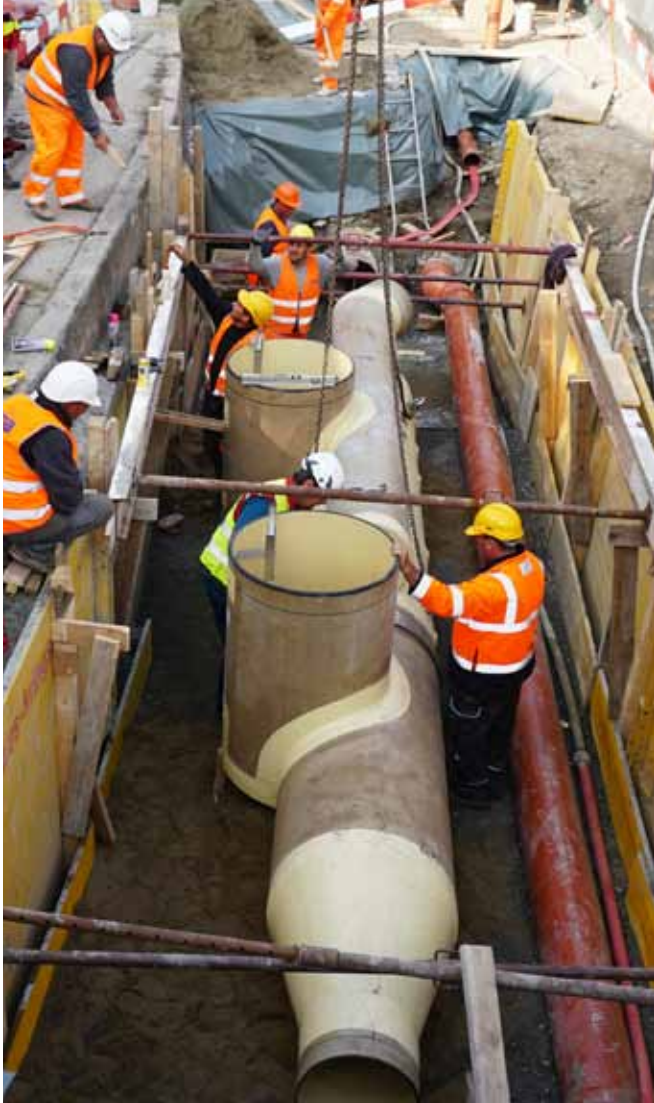
Top left: The CSO chamber was successfully installed in 1 day only. Bottom right: The highly effective and flexible cleaning elements (GRP bars). Top right: The project team did a great job and is pleased with the optimal result.
