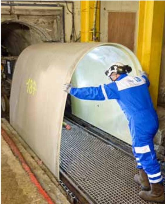
The NC pipes could be perfectly tailored to the customer's requirements and the technical specificities of the network. Following several preparatory works, the French construction specialist SADE started with the installation of the half-pipes on the channel's vault in November 2015. It can be accessed from four pits, from 40 to 105 meters deep, one of which is the Gabrielle's pit from where the half pipes are transported to be installed. Due to the narrow space on the storage area
