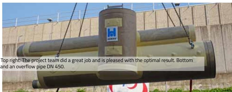
Left: The CSO chamber was successfully installed in 1 day only. Top right: The project team did a great job and is pleased with the optimal result. Bottom right: The modular CSO chamber with a GRP main pipe DN 800 and an overflow pipe DN 450.
