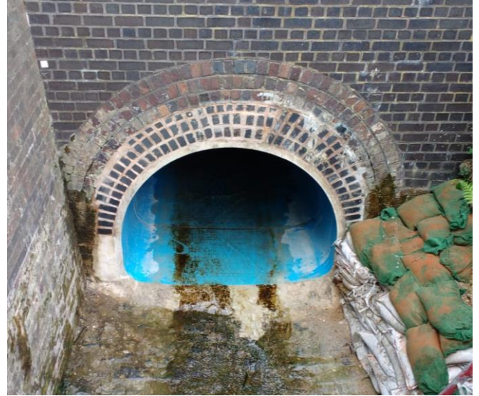
Culvert open and operational
