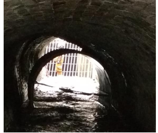
NC Line installation commenced (note deformation to culvert)
