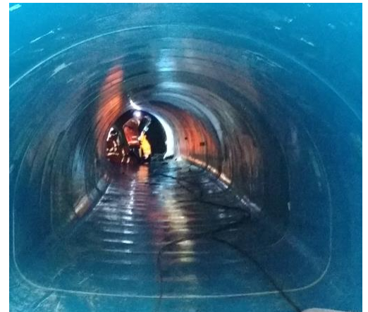
NC Line Installation negotiating a slight radius
