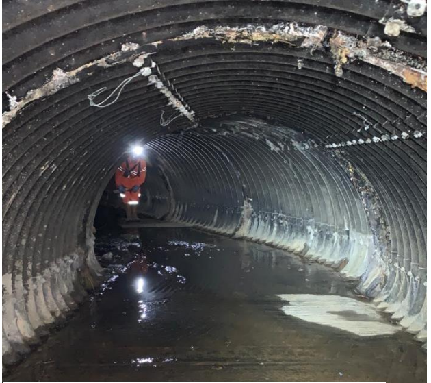
Fig 1: Host pipe inspection. Courtesy of MDA Ltd
