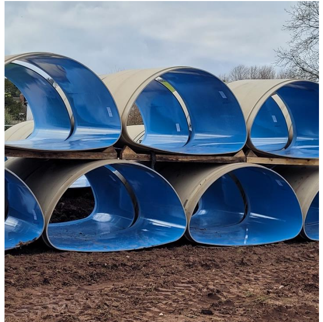
Fig 3: Amiblu NC Line 2360 x1350mm ready for installation
