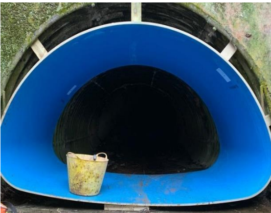
Fig 2: Site preparation. Courtesy of MDA Ltd
