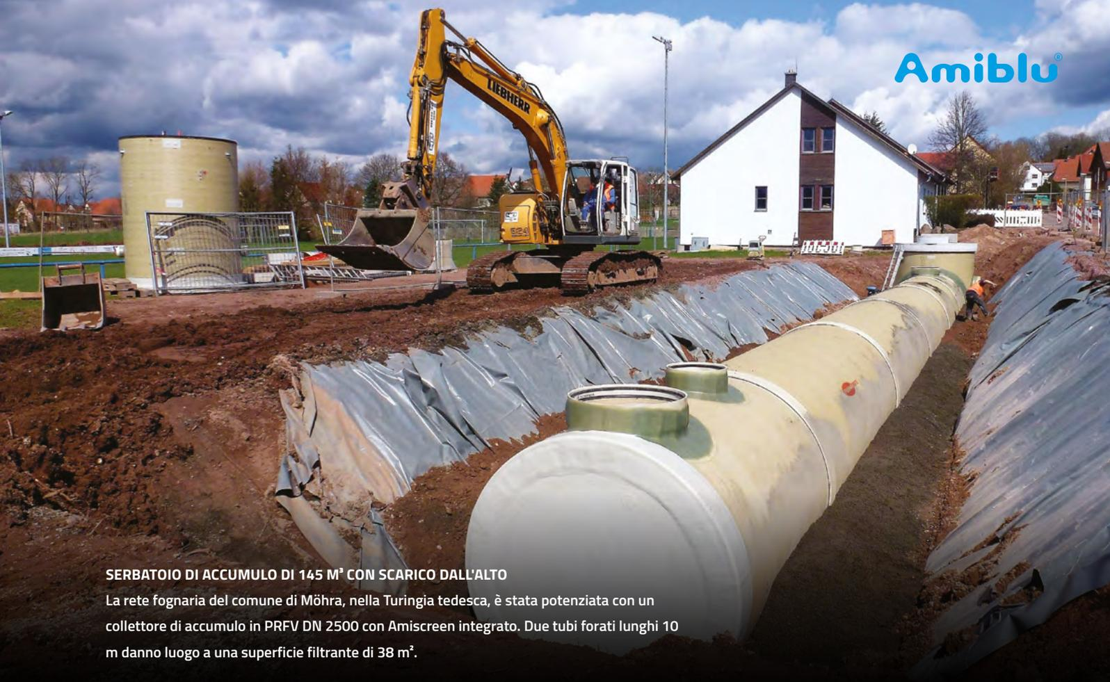
**SERBATOIO DI ACCUMULO DI 145 M<sup>3</sup> CON SCARICO DALL'ALTO**
