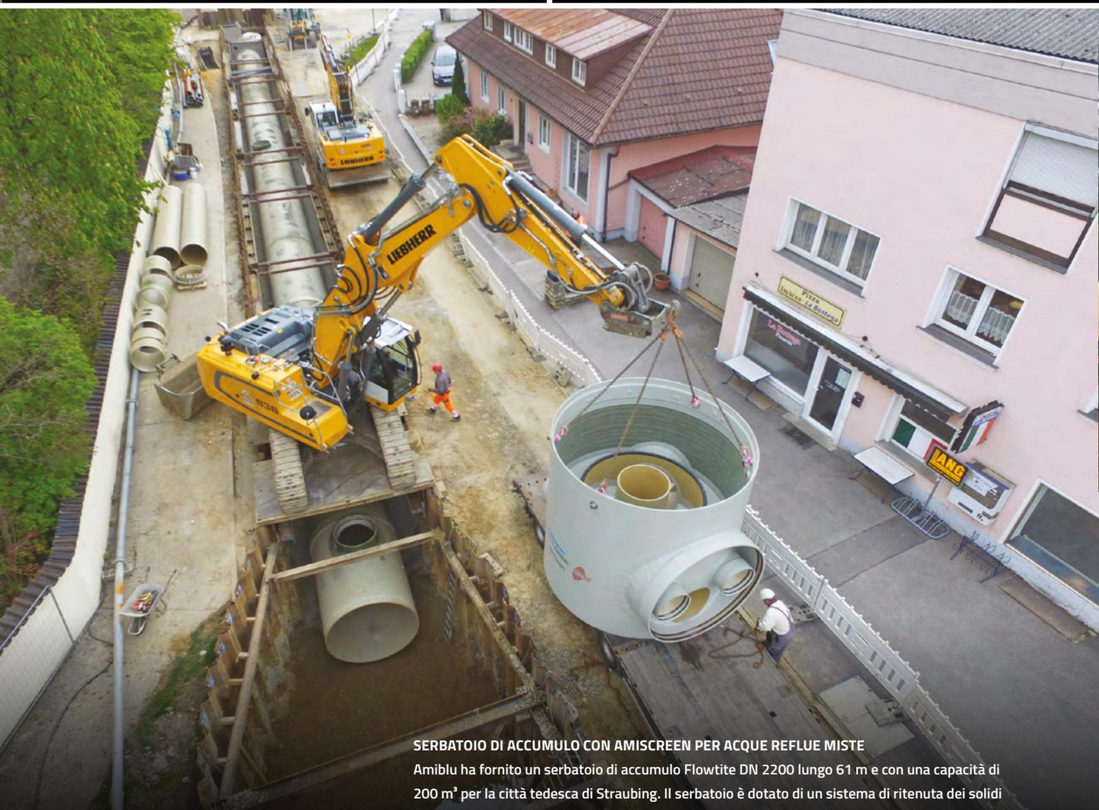
**SERBATOIO DI ACCUMULO CON AMISCREEN PER ACQUE REFLUE MISTE**
