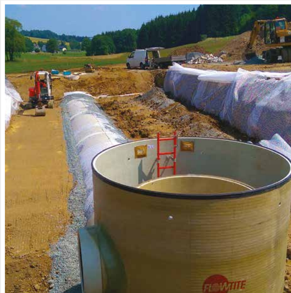
Stormwater overflow, trough inlet
