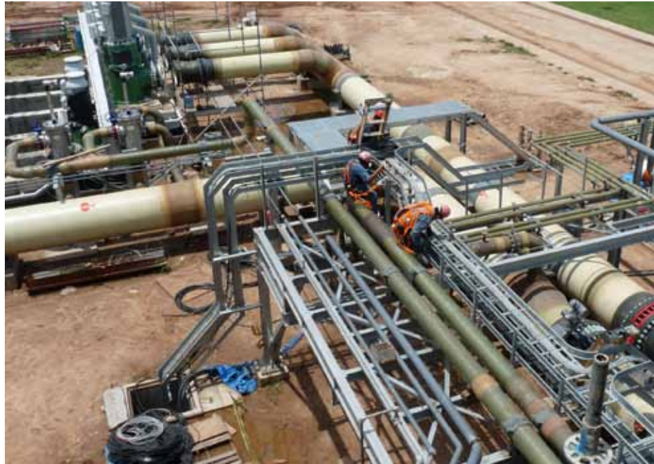
Amiblu supplied biaxial GRP pressure pipes DN 1000 and DN 700 as well as moulded biaxial pipes DN 25 to DN 250 (all Flowtite FW) for the two power plants.
