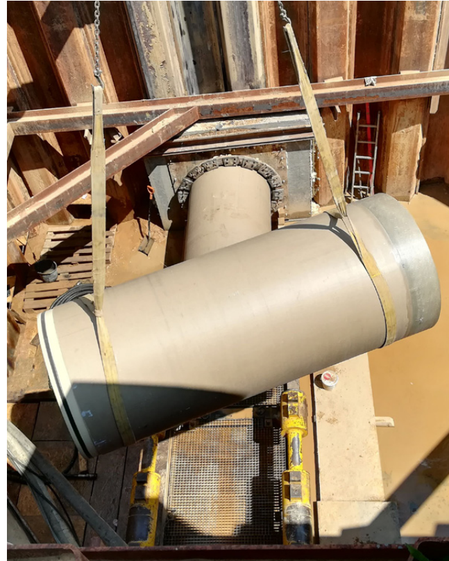
Top left: Flowtite pipes with distance rings were inserted into Hobas jacking pipes to create a highly sustainable and reliable pipe-in-pipe system. Top and bottom right: Hobas GRP pipes were used for microtunneling underneath roads.
