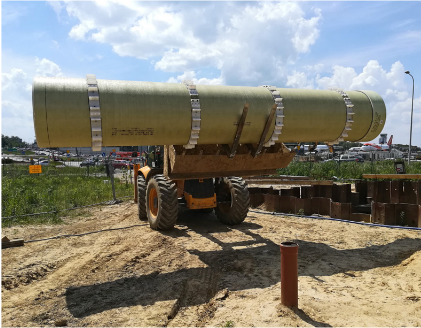
Top left: Flowtite pipes with distance rings were inserted into Hobas jacking pipes to create a highly sustainable and reliable pipe-in-pipe system. Top and bottom right: Hobas GRP pipes were used for microtunneling underneath roads.
