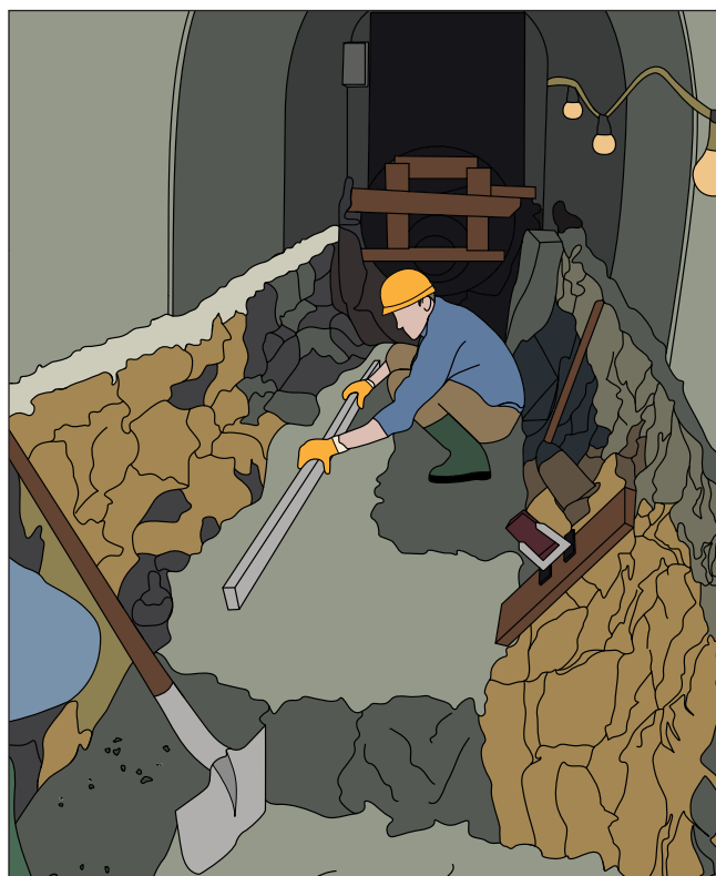
Fig. 17: Existing sewer bottom treatment for proper installation
