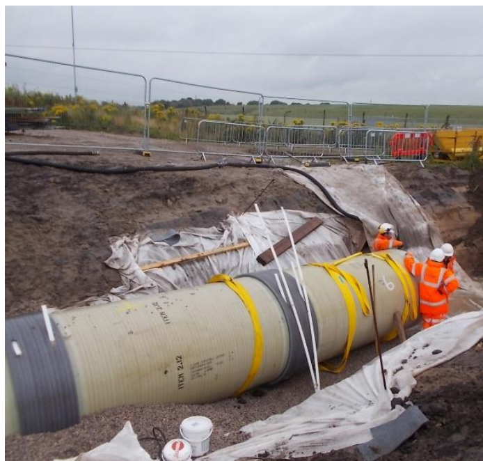
Fig 3: Flowtite Biaxial pipe c/w lock joint. Courtesy of MMB
