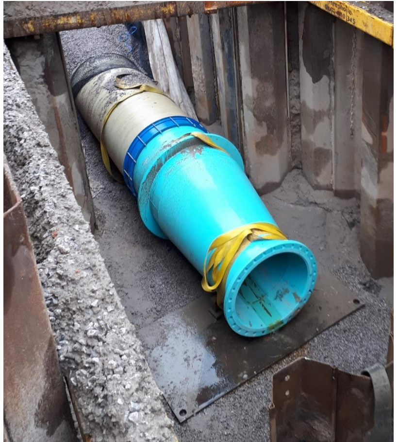
Fig 1: Laying new GRP pipeline Courtesy of MMB
