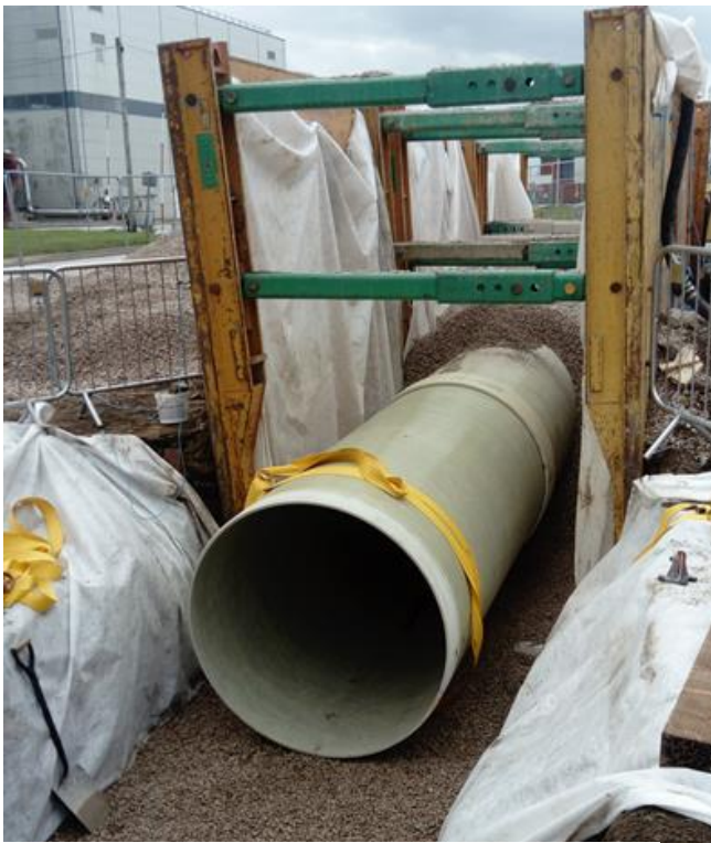
Fig 2: Laying new GRP pipeline Courtesy of MMB
