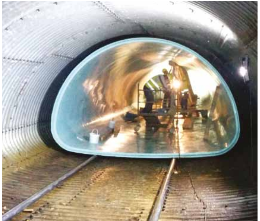
Top: Amiblu NC line pipes can be produced in all shapes and sizes to revive aged channels.
