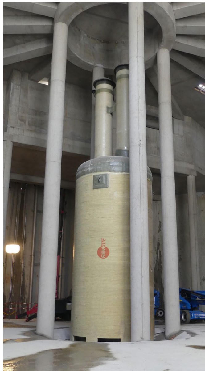
Above: A 7 m long vertical Flowtite pipe DN 3000 serves as flushing system inside the storage chamber.
