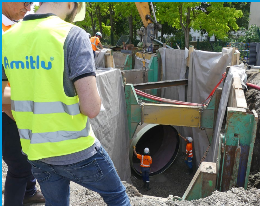
Right: A Hobas pipe system DN 2400 was installed between the intercepting chamber and the storage tank.
