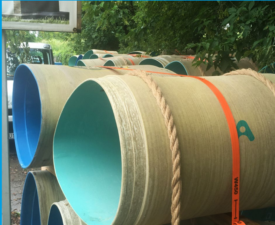
Above: 746 m of Amiblu NC Line pipes in various cross-sections were installed in the course of eight months to renovate parts of Krakow's aged sewer system.
