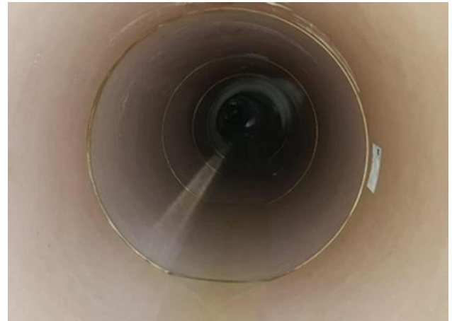
Fig 4: Courtesy of MDA Ltd. - installation complete
