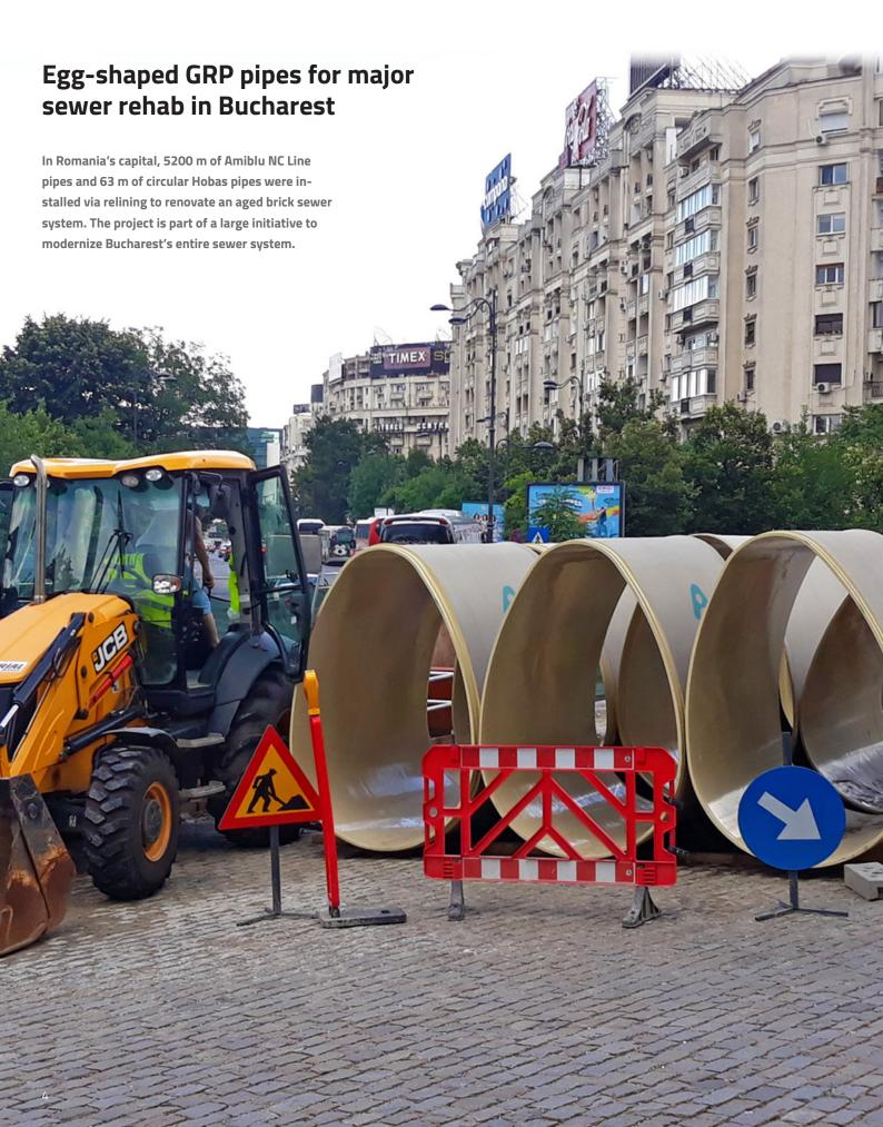
From 25 to more than 100 years: That's the fairly advanced age of the sewer system of the metropolis Bucharest. It was therefore decided to renovate the extensive system step by step in order to increase its efficiency and reliability. One of the sections to be rehabilitated is a particularly challenging one: near the Parliament house and old town, where space and accessibility are limited. Conditions that called for a special approach — and the perfect solution was found with Amiblu.
