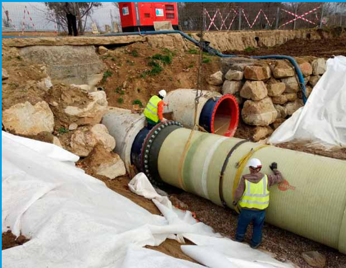
National regulations specified that two roads and one rail track were to be crossed with concrete jacking pipes and steel pipes. The steel and GRP pipes were then joined with a leak-proof flange connection.
