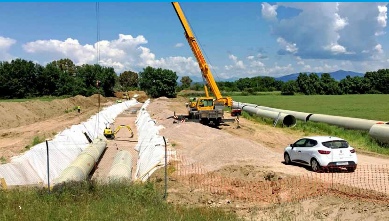
Bottom: Two GRP pipelines were installed to transport water from the Tagus River to the Lower Channel of Alberche.
