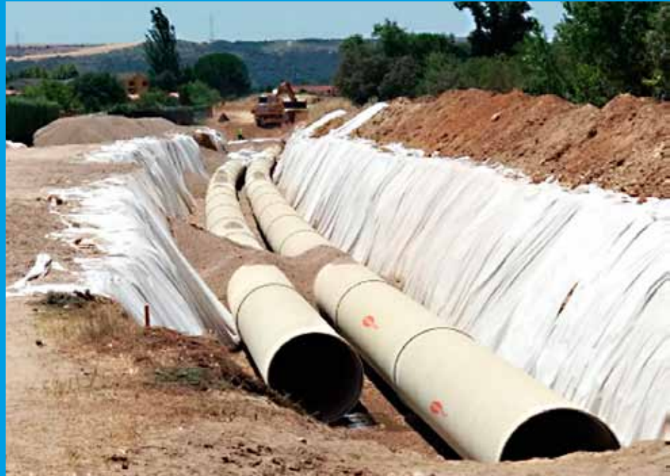
Top: Amiblu supplied 7.5 km of GRP pipes DN 1600 as well as multiple elbows and drains for the new irrigation system.
