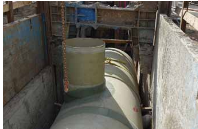
The new Flowtite storage sewer DN 2300 includes an intake and flow control shaft. The GRP solution outscored concrete in terms of durability, flexibility, and weight.
