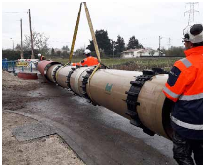
Bottom: GRP pipe DN 800 with distance rings.
