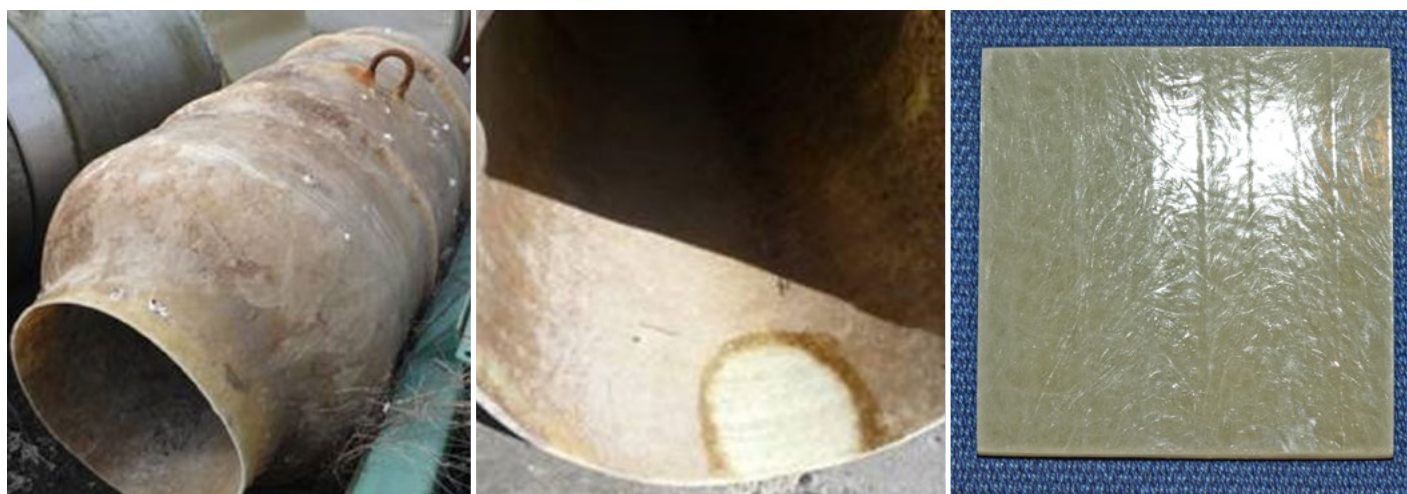
Fig. 11-13: In 2008, after 33 years exposure to treated sewer and seawater, a section of a Flowtite GRP DN 500 pipe was brought ashore for analysis of its condition and mechanical properties. After cleaning parts of it, the pipe looked almost brand-new. The pipe showed no visible signs of ageing and its mechanical properties were basically unchanged.
