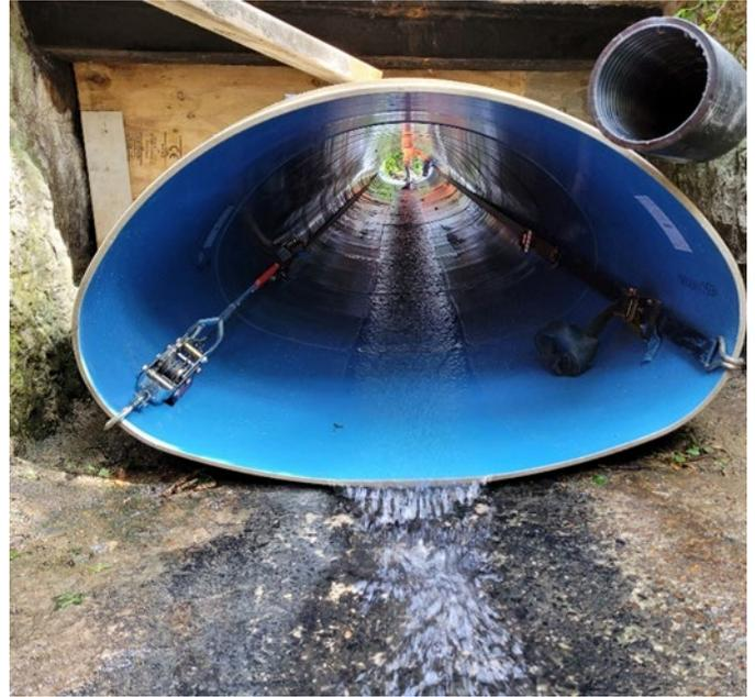
Fig 3: Amiblu NC Line Installation courtesy of Steadline Ltd
