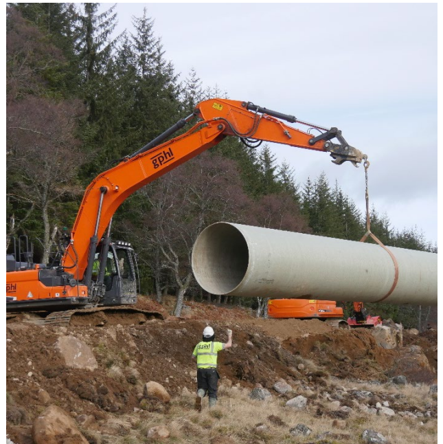
Fig 3: DN1600 PN10 Flowtite Pipe – courtesy of GPHL
