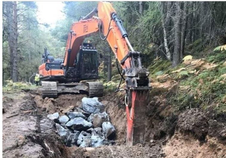
Fig 2: Site preparation. Courtesy of GPHL
