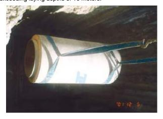
The ground conditions were very poor and soil consisted of layered mudstone, gypsum and sandy-silt with a high ground water table. The total project was divided into several contracts, whereas the biggest part was realized by the local firm. This section consisted of approx. 24 km in a diameter range of DN 400 to 1800 and HOBAS received the order to
