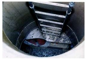
Then the old pipe in each entry shaft was cut open lengthwise and used as an insertion guide for the new liner pipes. Pipes were simply driven through manholes that were no longer required; manholes at pipeline bends were replaced with smaller HOBAS Bends or rehabilitated using HOBAS GRP.
