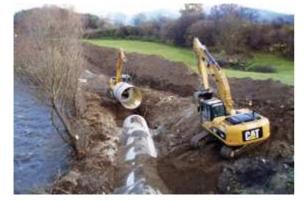
HOBAS CC-GRP Pipe Systems easily fulfilled all requirements. Since October 2008, HOBAS Pipe Austria has been delivering the unique HOBAS CC-GRP Pressure Pipe Systems including FW couplings to the new power plant Penz VAEE, which is operated by Mr. Rochus Penz, VAEE and the constructor Zotter.
