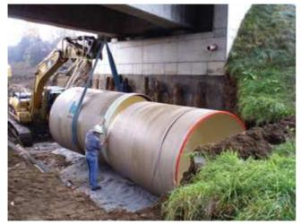
The pipeline is installed in three phases, leading from the power plant Penz to the estuary of the rivers Pöls and Mur and finally to the power house on VAEE property.
