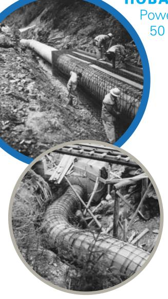
Today, almost half a century later, the hydropower plant Filisur is still in operation. Together with the plant Tiefencastel it produces around 381 million kWh which approximates 5 % of the annually produced electricity in Grisons. Over the years, the GRP pipes have been regularly inspected and have been reliably doing their job ever since the plant's startup.
