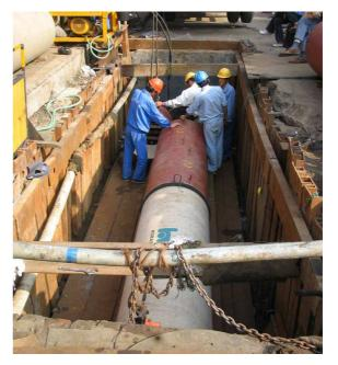
CC-GRP Jacking Pipes with steel collars were chosen as the best solution. The requirements regarding pipe design are: HOBAS Pipes with an outer diameter of 800 mm, SN 5000, PN 8. The roughness coefficient of the inner surface is 0.009 - 0.01. Given the data above, calculations showed that the flow capacity of the HOBAS<sup>®</sup> CC-GRP Pipe DN 800 was similar to that of the DN 900 cast iron pipe.
