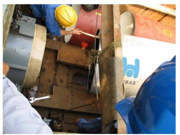
The installation was started in October 2006. Starting and receiving pits were established at suitable locations along the course of the sewer. The old cast iron pipe was cleaned and working platforms were installed. Then about 1163 m of DN 800 HOBAS<sup>®</sup> CC-GRP Pipes were
