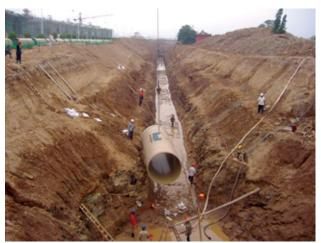
Several reasons let the municipality Yiwu decide for HOBAS centrifugally cast, glass fiber reinforced pipe systems. The mentioned weak soil conditions, for instance, would have made the use of heavy equipment elaborate. However, CC-GRP pipes weigh a lot less than other materials and are
