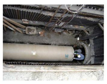
All rehabilitation work on the canal was done from the existing shafts or from the operating pipe shaft. Due to the work in the canal, the inlet and outlet had to be closed and the water had to be pumped out. In the whole section, solid sediments on the bottom of the pipe and the chambers were removed and at the same time deposits under the shafts
