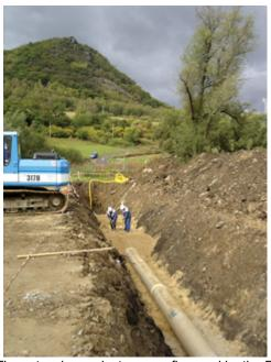
The extension project was co-financed by the EU program ISPA and involved the reconstruction of a part of the existing DN 600 potable water main running along the same railway track and from the highway to the river Bilina. All in all 5.7 km of HOBAS CC-GRP WaterLine® Systems DN 500, PN 16, SN 10000 were utilized for the project that was completed in 2006.
