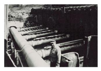
From 1981 through 1984, pipes were installed in several stages for disposing of the effluent and conveying it to the wastewater treatment plant. A total of 14 km of HOBAS Pipes were used here and installed by open trench construction as well as above ground. Particularly interesting is the part of the line laid above ground. Its route includes a pipeline bridge over the River Ostravice and takes the industrial wastewater to the company's treatment plant and a reservoir.
