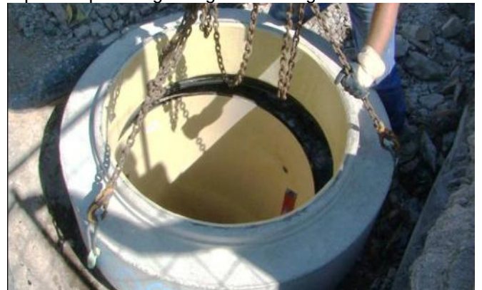
DE09SHL_Schockwitz 4: Fitting a concrete cone onto the shaft
