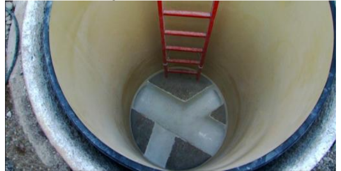
DE09SHL_Schockwitz 3: Minimal loss in cross-section
