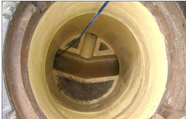
DE09SHL_Salmuende 5: The GRP lining perfectly seals the old shaft
