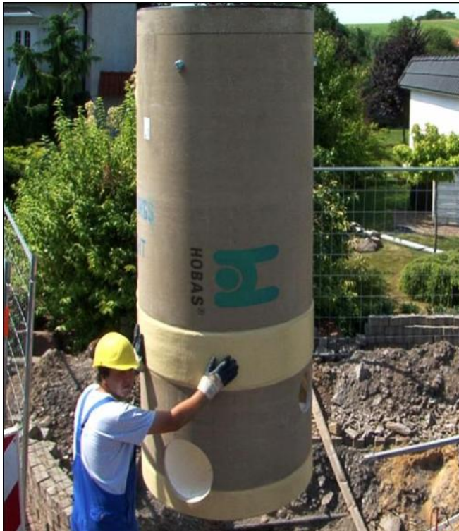
DE09SHL_Schockwitz 1: New GRP Shaft lowered into existing shaft
