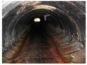
After a collapse of structures in 2004, the Ministry of Equipment & Transportation decided to secure the most critical ones. One third of the steel constructions (corrugated galvanized steel culverts) and a number of concrete culverts had visible defects. Nearly half of these culverts were in poor condition and required full rehabilitation as soon as possible.
