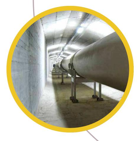
for it minimizes the number of necessary supports. Easily jointed pushto-fit couplings contributed to the savings since no welding is required for HOBAS Products.
