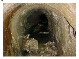
Turin, Italy has a network of sewer pipelines which comes from the ancient time. It is estimated that more than 80% of these pipelines are egg-shaped; even today, most of the new ones are made with egg-shaped concrete pipes.
