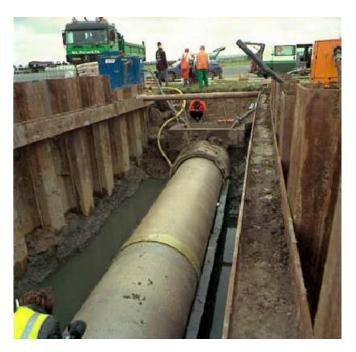
The Schiphol group is now using HOBAS<sup>®</sup> CC-GRP Pipe Systems with stiffness of SN 16000 or higher for more renovation projects as well as for new pipelines, the reason being the high operational life time of HOBAS<sup>®</sup> Products and the high statical loads occurring on air fields.
