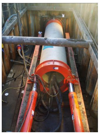
Preparations for jacking commenced in January 2010 so that it was likely that there would be no more frost by the time the jacking pits and equipment were ready. Temperatures, however, fell again and halting construction works was not an option. Since CC-GRP Pipes are insensitive to extremely low (and high) ambient temperatures the challenge lay in
