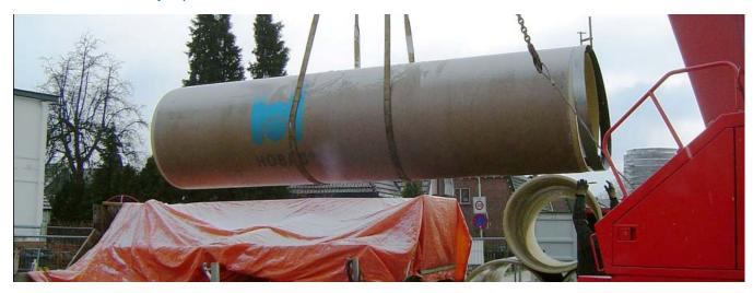
Despite the extremely frosty temperatures (-15° C) during construction works at the beginning of the year 2010, the municipality Doetinchem in the Netherlands was able to complete the extension of its overloaded sewer main with HOBAS CC-GRP Jacking Pipes. The round 57,000 inhabitants can now count on a flood-free sewer for at least five decades.
