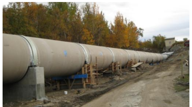
NO08HYL_Helleren 5 - Casting the pipe supports on precast base
