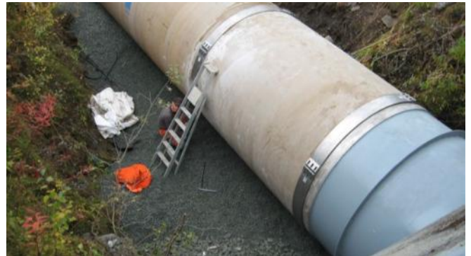
NO08HYL_Hellen 7 - Assembly of pipeline to steel intake with mechanical coupling
