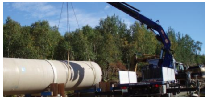
NO08HYL_Helleren 4 - Pipes being delivered directly to the supports on site
