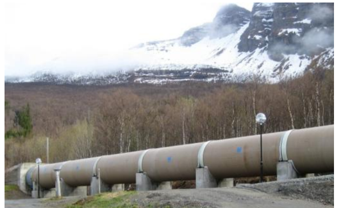
NO08HYL_Hellen 7 - Assembly of pipeline to steel intake with mechanical coupling
