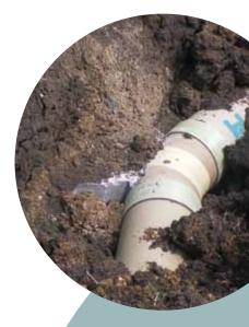
Year of Construction 2009 Total Length of Pipe ~ 2.1 km Pipe Specifics PN 6, SN 5000, DN 500 Installation Open trench Application
