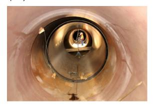
The Water Company of Bratislava, who was in charge of finding the optimal solution to the results of revaluation, decided to reconstruct and to extend the existing waste water system. They proposed to have the old DN 2600/1650 concrete pipeline cleaned and recommended its rehabilitation with HOBAS® CC-GRP SewerLine® Systems DN 1400. HOBAS products were chosen due to their hydraulic performance, the proven leak tightness of the system and the relatively low weight of even large profiles.
