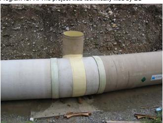
experts and redesigned to utilize HOBAS CC-GRP HOBAS<sup>®</sup> SewerLine<sup>®</sup> DN 1800 Pipes SN 5000. Decisive criteria were leak-tightness, durability, hydraulic and long-term static characteristics as well as numerous similar reference projects involving similar constructions to demonstrate the experience of HOBAS in the field.
