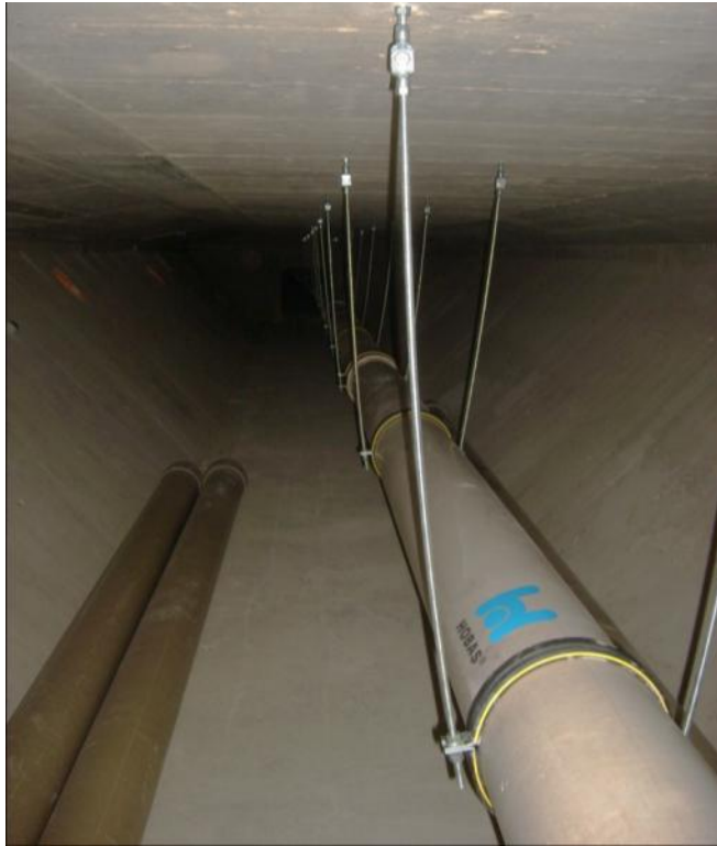
SK10BRL 3: HOBAS Pipe installed in the bridge
