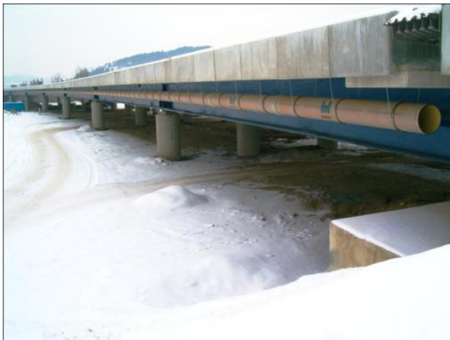
SK10BRL 1: HOBAS BridgeLine Pipes fixed on hangers
